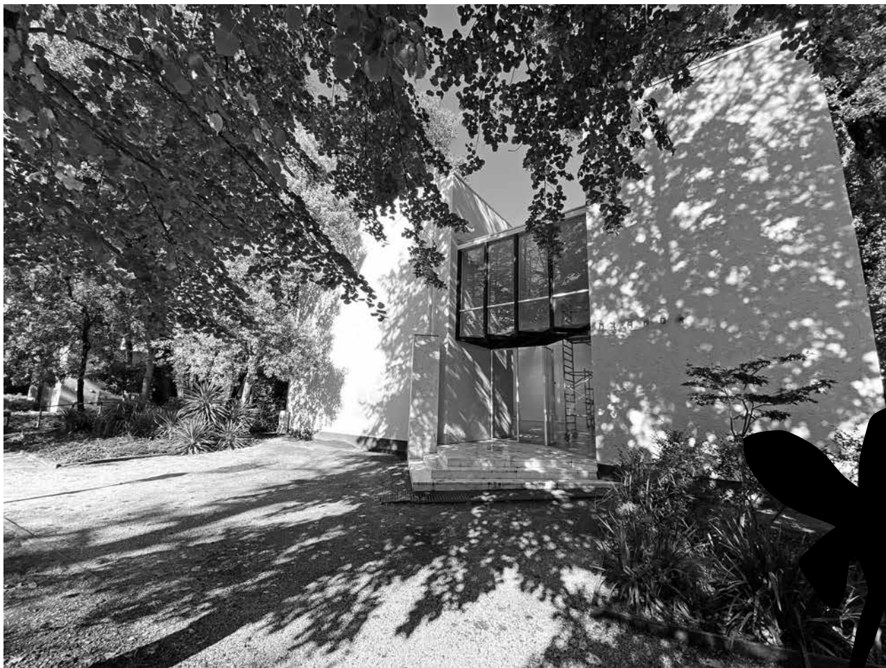
Rietveld Pavilion in 2021. Photo: Corina L. Apostol.
